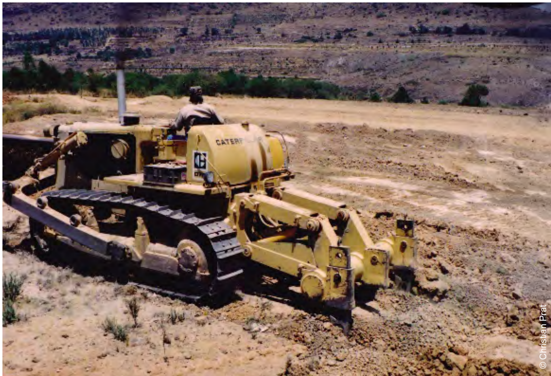
Photo 79. Heavy machinery breaking
