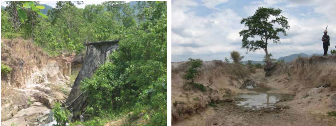
Figure 7: Dyke (left) and Channel (right) Constructed During the Khmer Rouge Era (1975-1979)
